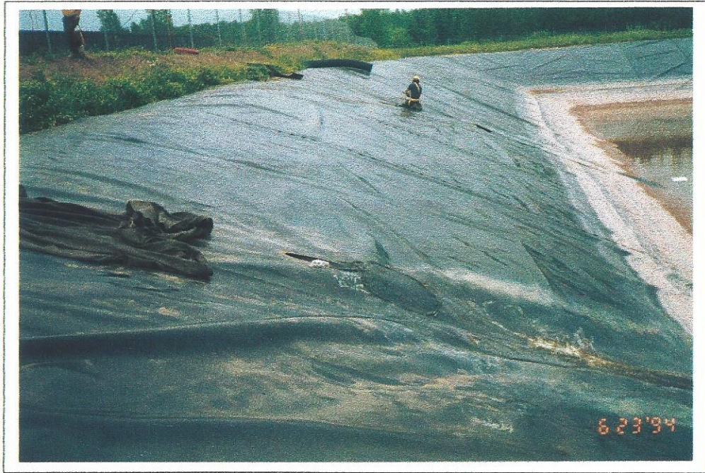
#7 PROFILE OF COMPLETED REPAIR
