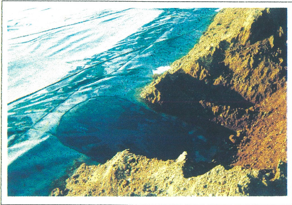
STOCKPILE II PHASE I HDPE LINER LOCATION 2 OF 3 REPAIR (TYPICAL)
