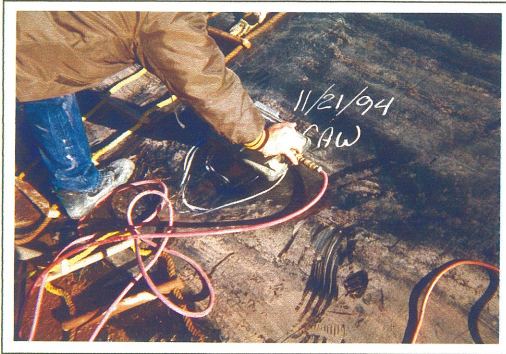
TYPICAL VACUUM BOX TEST REPAIRS #7-#10 11/21/94
