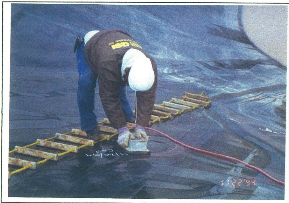
TYPICAL VACUUM BOX TEST REPAIRS #1-#6 11/20/94
