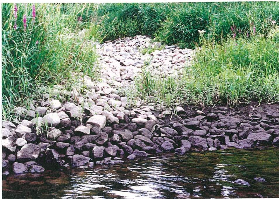
Photograph 2 August 1994 Flambeau River at Flambeau Mining Company outfall 002. Note no sediment from outfall but some deposition from action of river washing sediment across the mouth of outfall.
