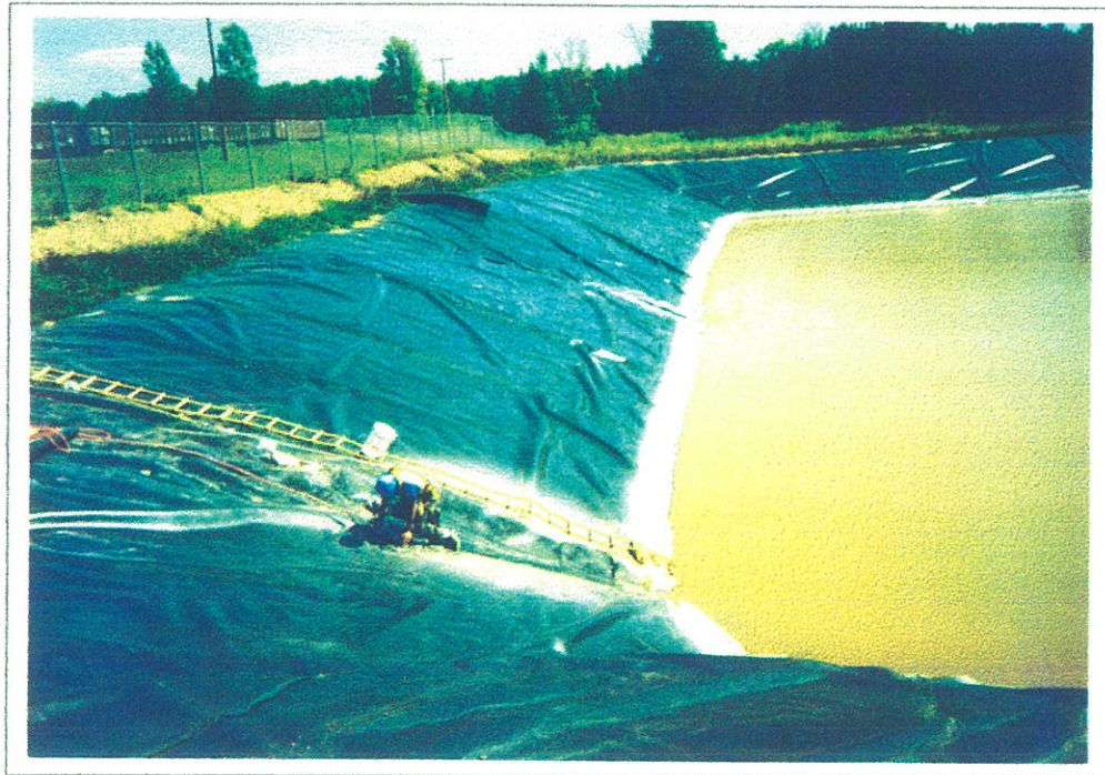
SURGE POND DISCHARGE PIPE HDPE LINER MODIFICATION SEAM TESTING
