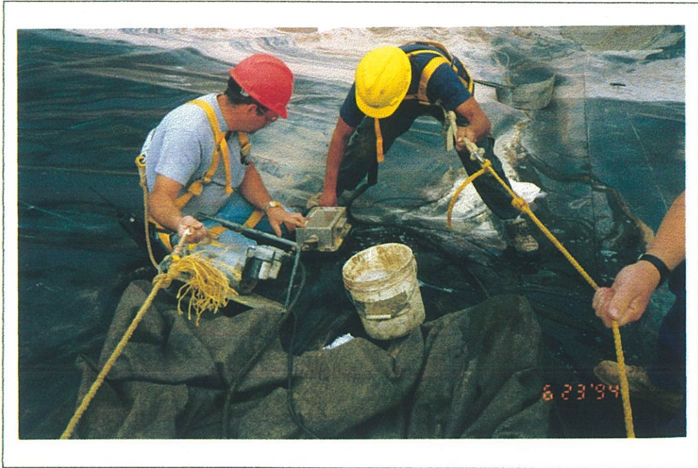
#5 PATCHING AND TESTING
