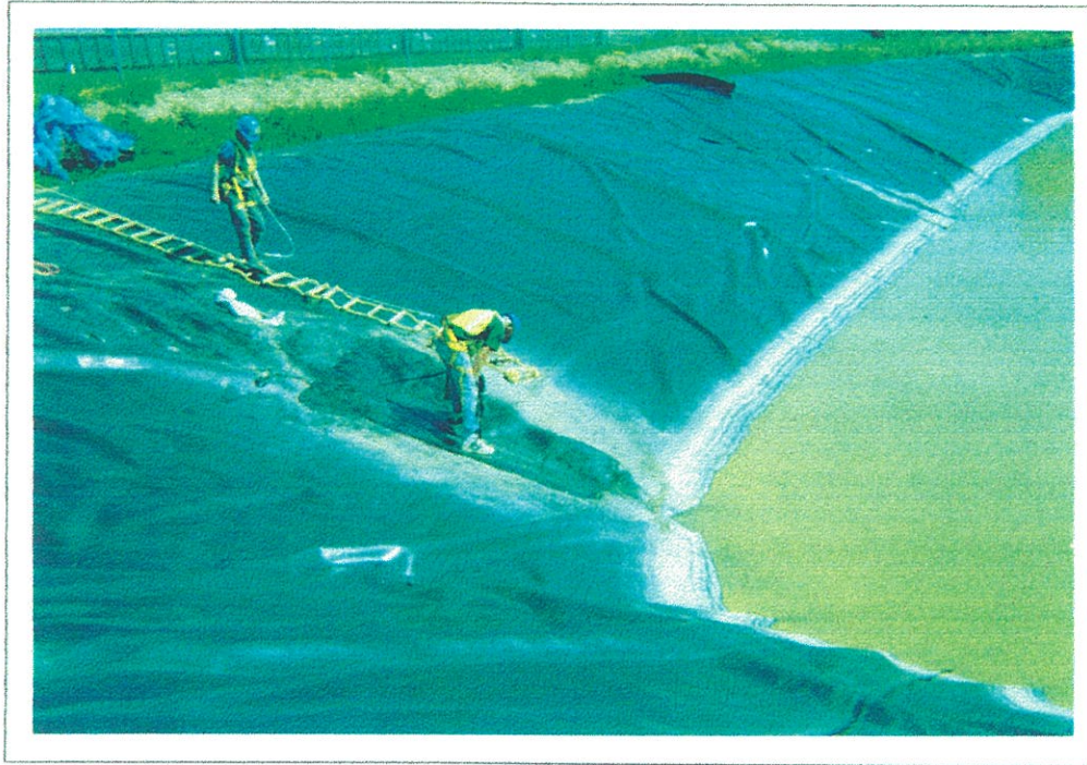
SURGE POND DISCHARGE PIPE HDPE LINER MODIFICATION
