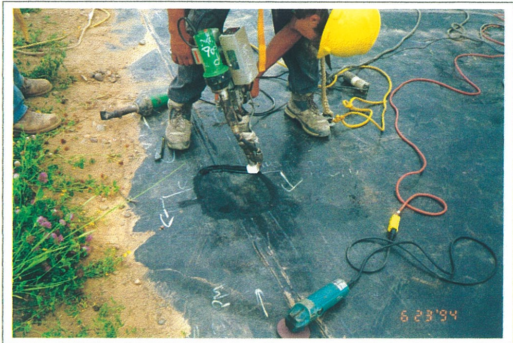
#2 TYPICAL PUNCTURE PATCH
