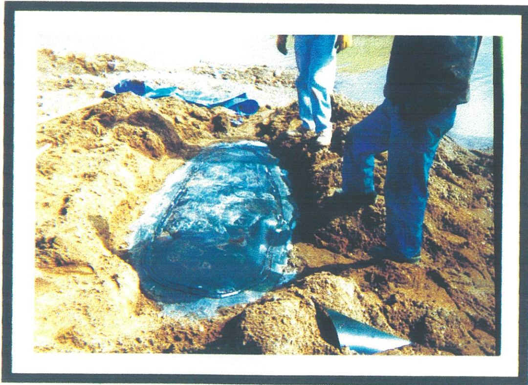
TYPE II STOCKPILE PHASE II LINER REPAIR MARCH 21, 1995
