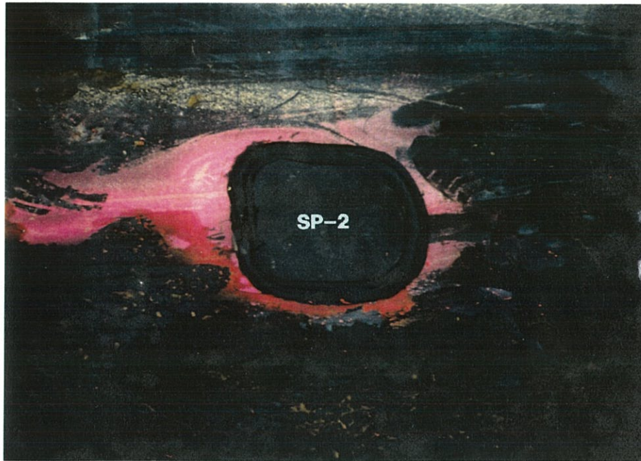
Photograph 5 October 9, 1995 Location: Surge Pond Liner-Repair Description: Repaired Puncture SP-2
