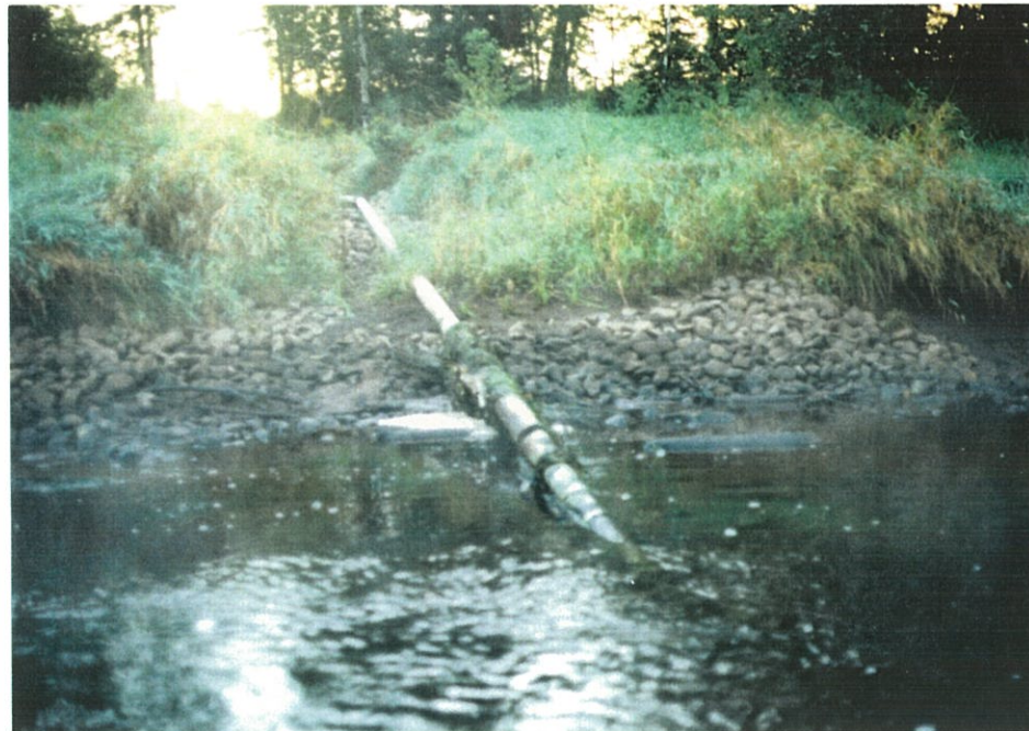
Photograph 2 September 1995 Mine discharge channel outfall 002 with temporary intake pipe for hydic soil recharge and emergency dust suppression in-place.
