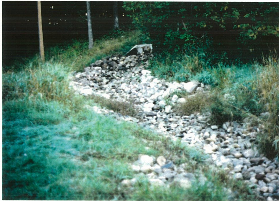
Photograph 3 September 1995 Outfall 001 showing no signs of deposition of sediments from the discharge of treated effluent.
