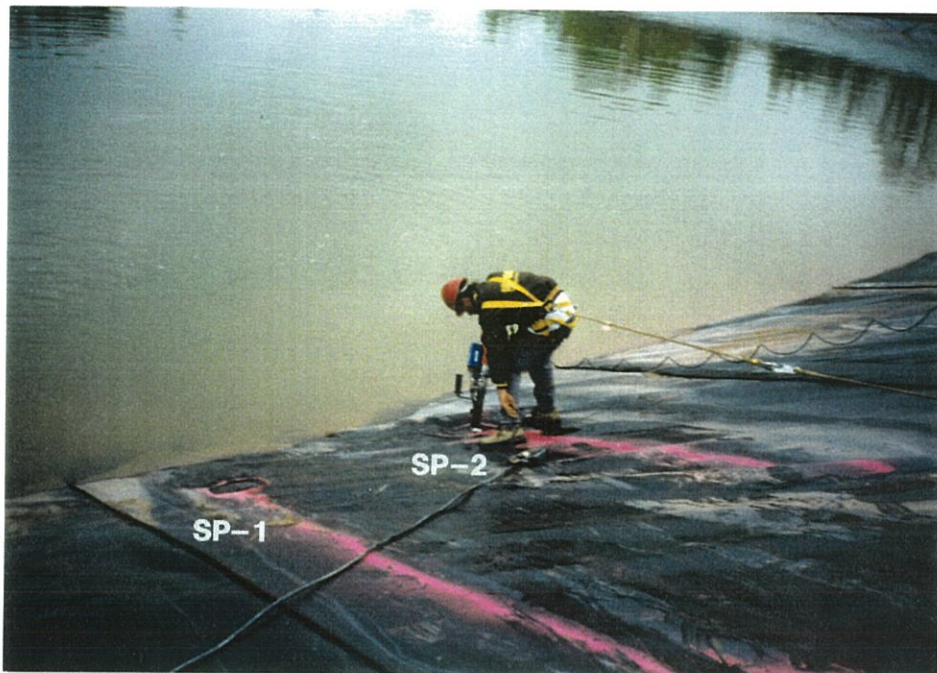
Photograph 3 October 9, 1995 Location: Surge Pond Liner-Repair Description: Extrusion welding repair SP-2
