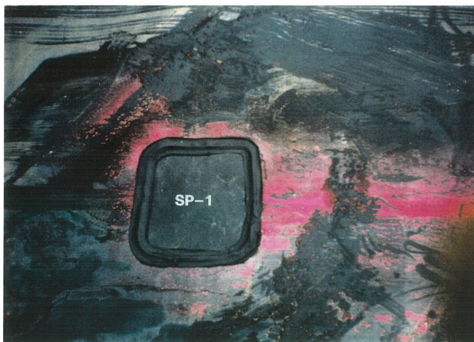
Photograph 4 October 9, 1995 Location: Surge Pond Liner-Repair Description: Repaired Puncture SP-1.
