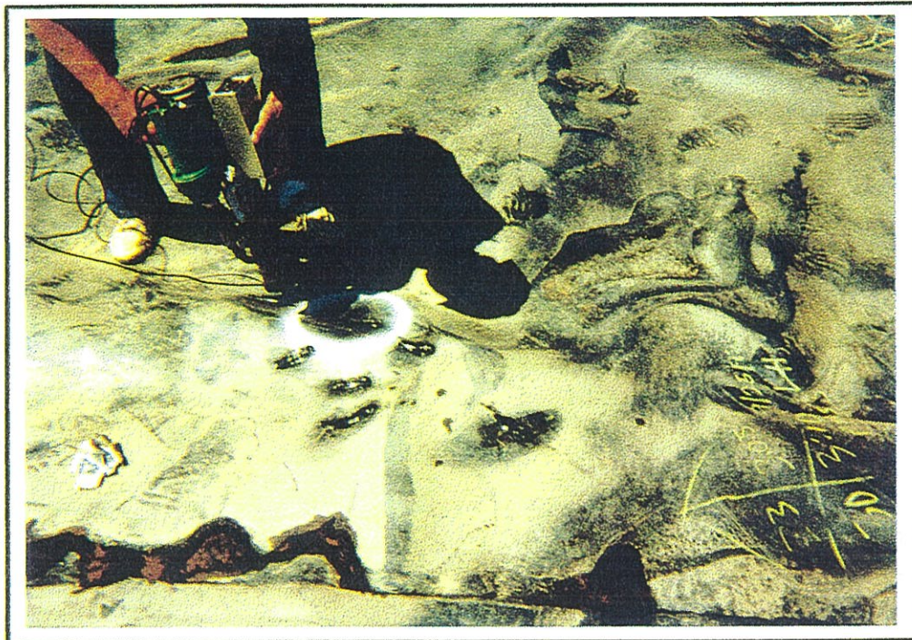
TYPICAL WELD REPAIR
