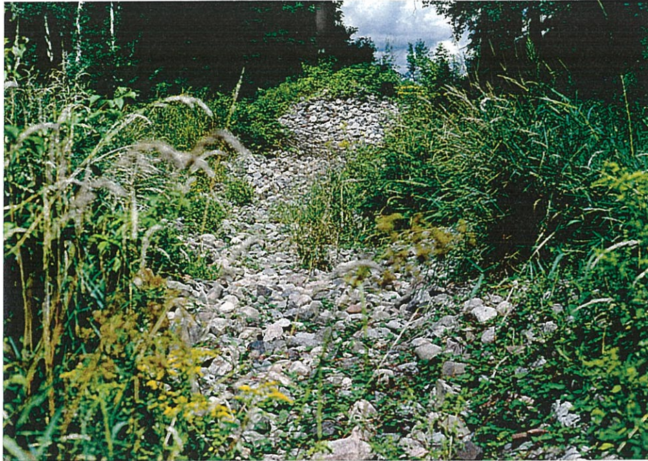
Photograph 1: View of Upstream Portion of Outfall 002
