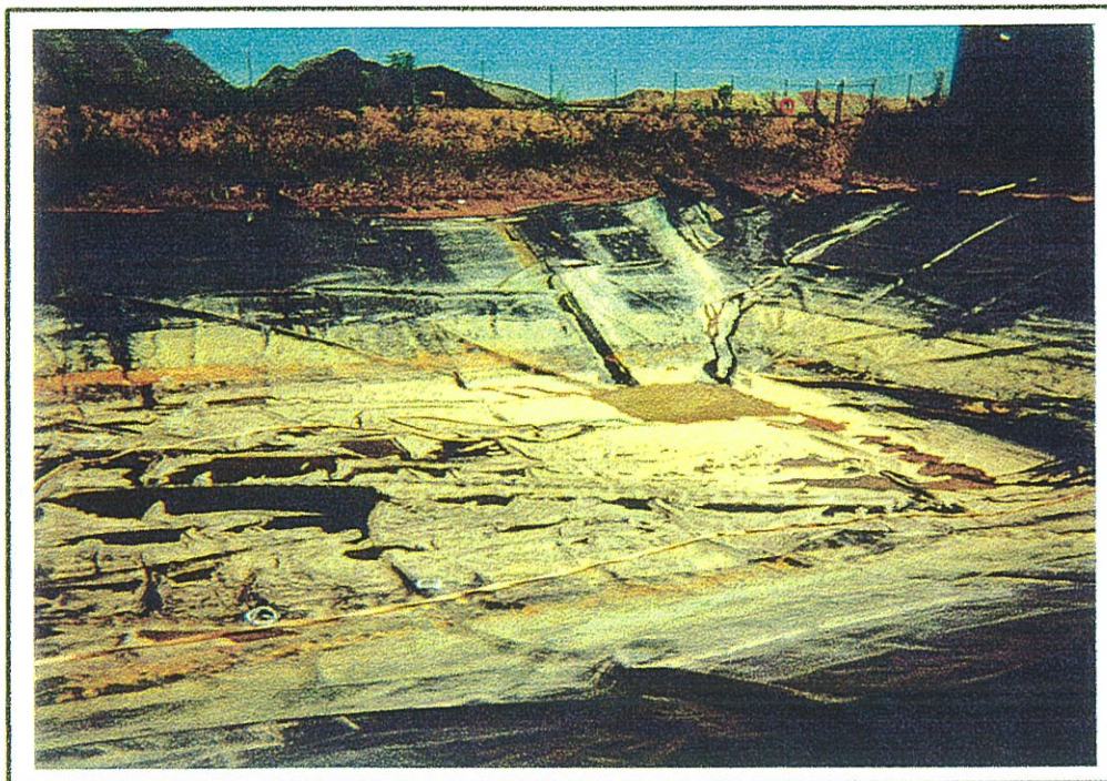
CAMERA LOOKING EAST
