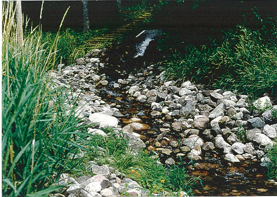
Photograph 3: View of Outfall 001 Looking Upstream at Origin of Outfall
