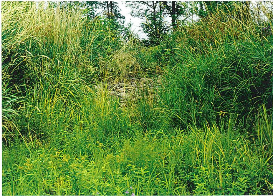
Photograph 1: View of Downstream Portion of Outfall 002
