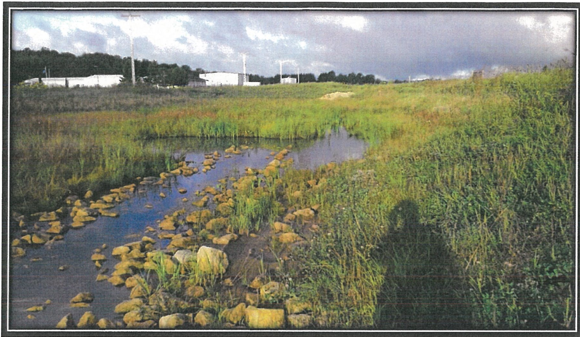
Photograph 15. North Area looking west with naturalized low flow channel and rock-lined swale, September 8, 2016.
