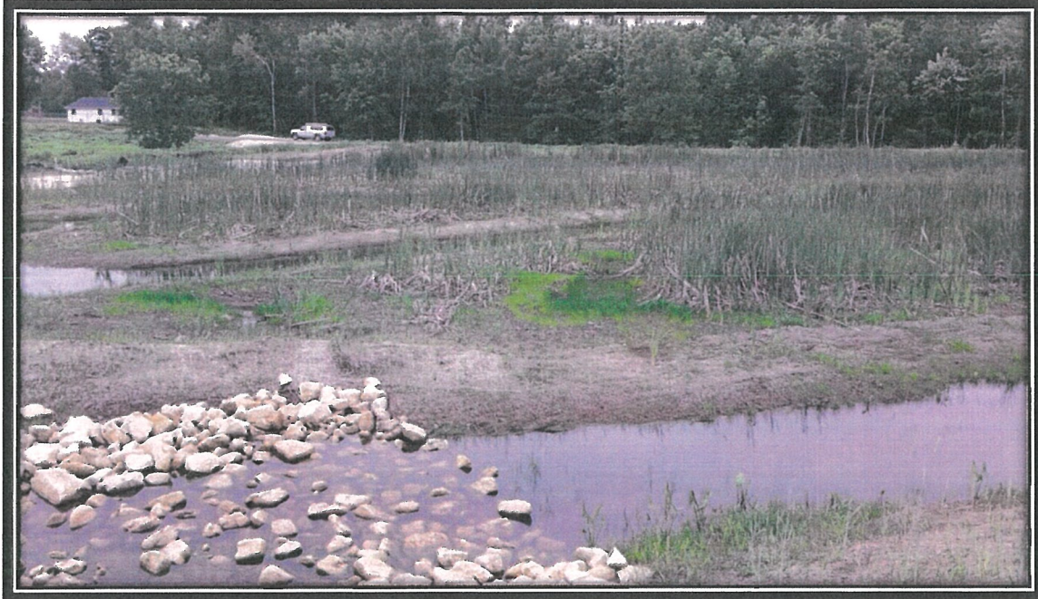
Photograph 5. East Area and naturalized low flow channel with initial seed germination on June 16, 2016. Erosion blanket is still intact.
