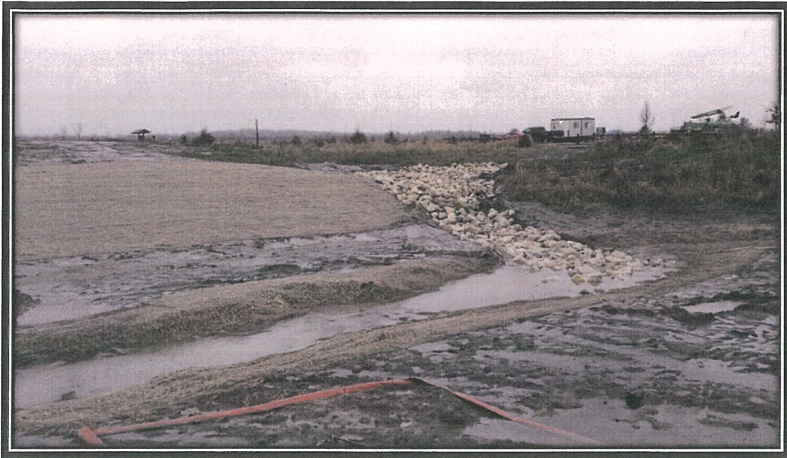
Photo 17. Surface water inlet in the northwestern corner of North Area with rock rip rap and side slope with erosion blanket in November, 2015.
