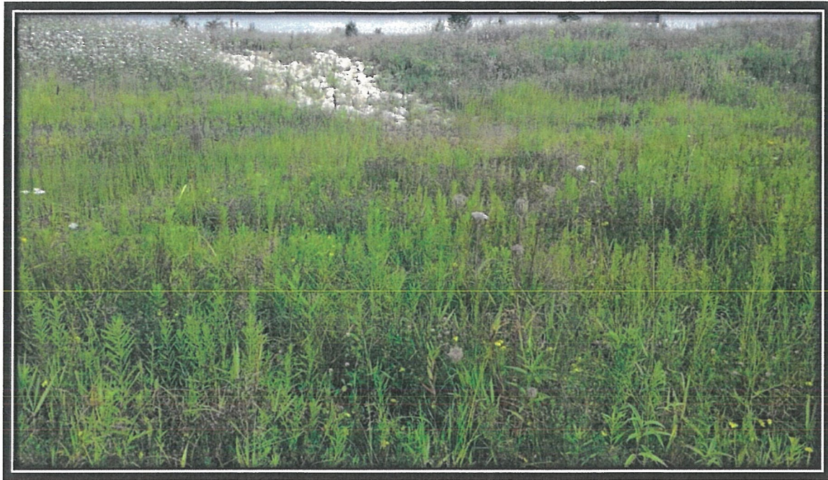
Photograph 19. Surface water inlet in the northwestern corner of North Area with rock rip rap, August 9, 2017.
