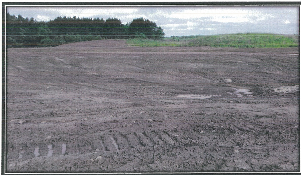
Photograph 26. Final grading of the West Area on June 16, 2016.
