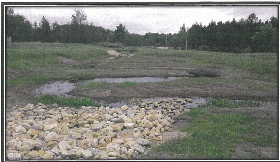
Photograph 11. North Area low flow channel looking east on June 16, 2016.
