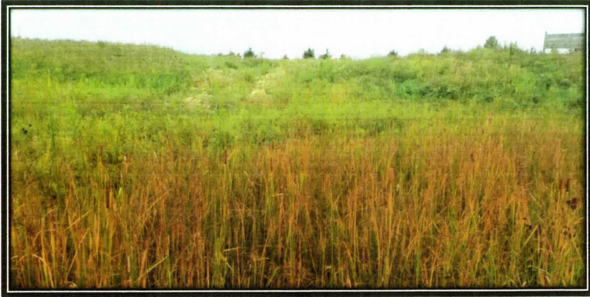
Photograph 24. Surface water inlet in the northwestern corner of North Area with rock rip rap on August 29, 2018.
