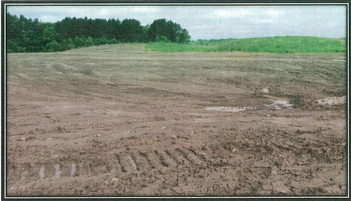
Photograph 34. Final grading of the West Area on June 16, 2016.
