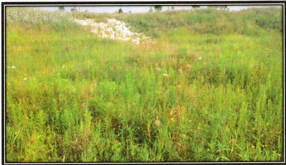
Photograph 23. Surface water inlet in the northwestern corner of North Area with rock rip rap, August 9, 2017.
