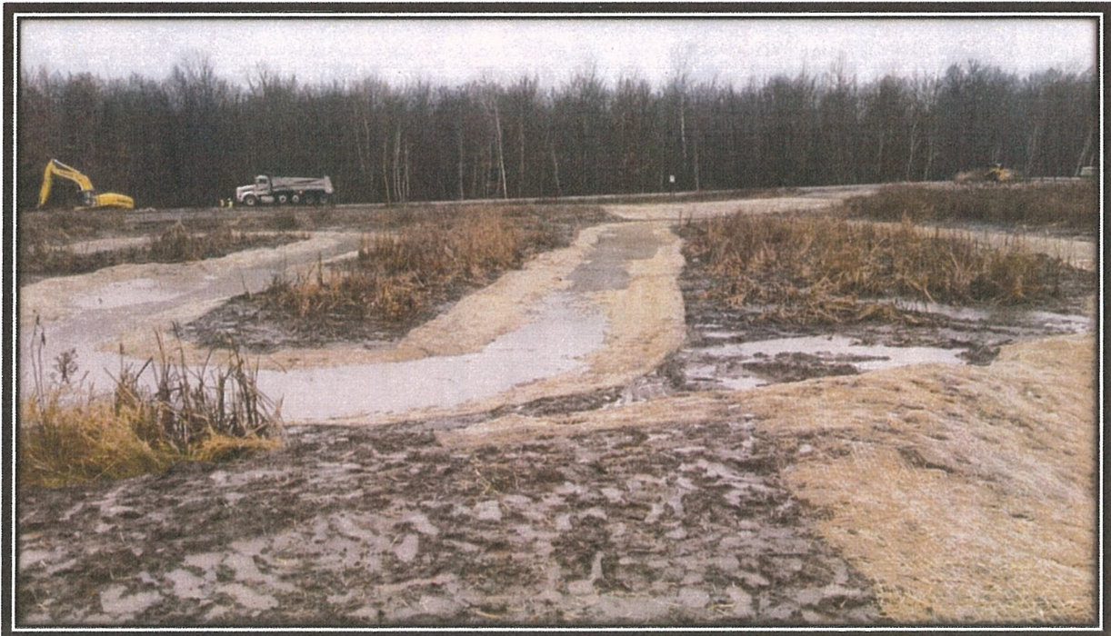
Photograph 2. East Area naturalized low flow channel with erosion blanket on November 17, 2015.
