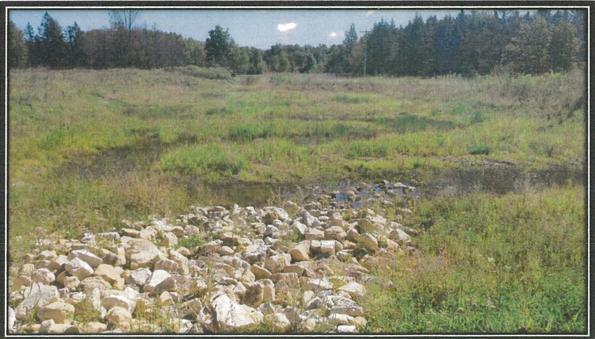
Photograph 14. North Area naturalized low flow channel (S shaped depression) amongst wet meadow "fingers" in September, 2016.
