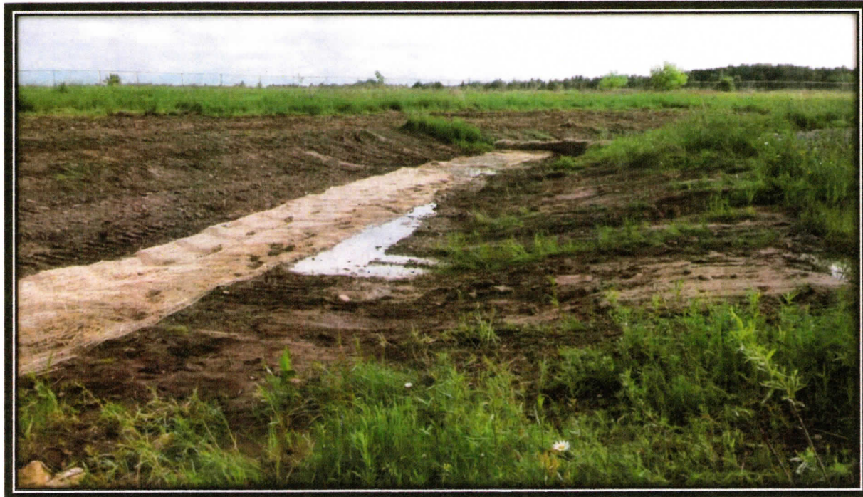
Photograph 28. East-West Swale final shaping and erosion control blanket in place along the swale on June 16, 2016.
