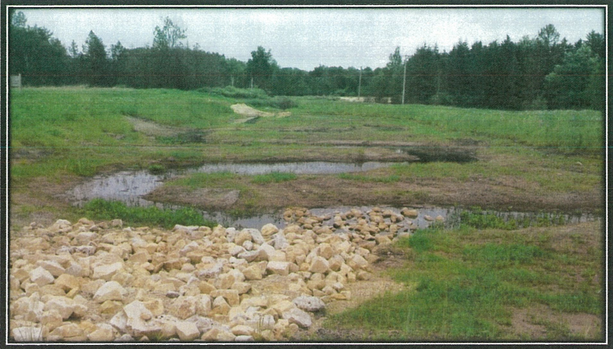
Photograph 13. North Area low flow channel looking east on June 16, 2016.
