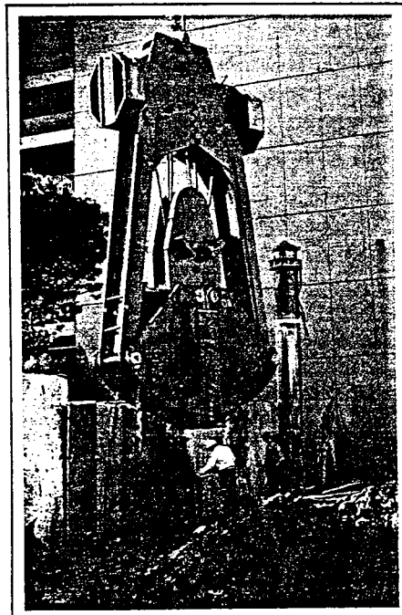
Slurry clamshell shown excavating secondary panel.
