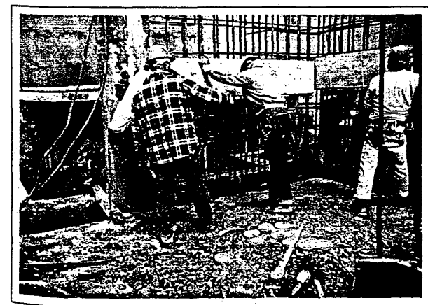
▲ Placement of corner steel reinforcing cage.
