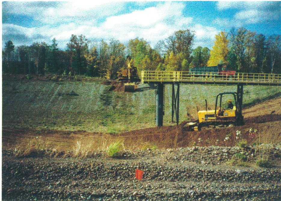
Photograph 2 October 5, 1995 Location: South Pond Description: Removal of Rip-Rap and vegetation.
