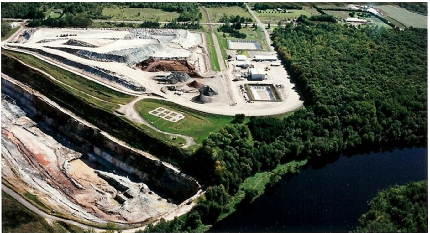
Figure 3. Top photo shows FMC waste water treatment plant, runoff pond, surge pond and other mine features, including the “high” sulfur waste rock stockpile and crushed ore storage area. Bottom photo shows the Flambeau Mine pit and nearby Flambeau River (1995).
